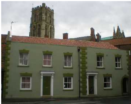
Quoin detail on 66 Bridgegate
