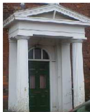
Doric pediment doorcase at 41 Hailgate
