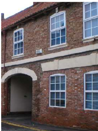
Painted string course shown below the first floor windows on Bridgegate.
