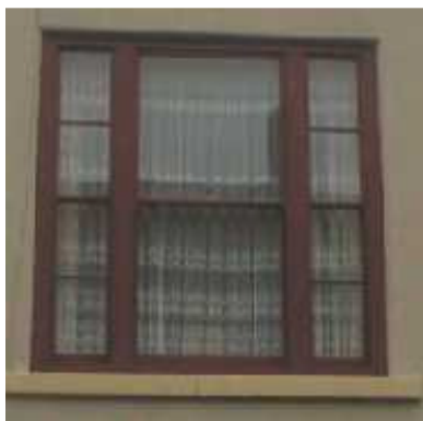
Tripartite window at No 73 Hailgate
