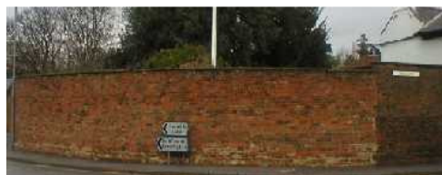
Boundary wall at Howden Hall, Station Road
