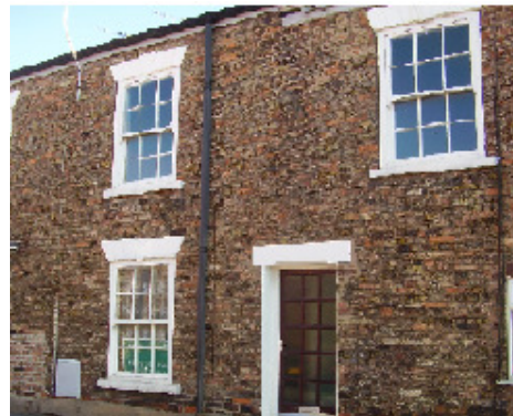
Flat arch lintels on Bishopgate
