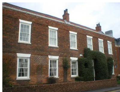
Parapet visible on No 15 Bridgegate House, Bridgegate
